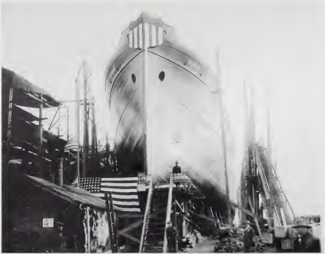
First Ferris-type ship built by Wilson Shipbuilding, the Quoque, launched May 18, 1918
