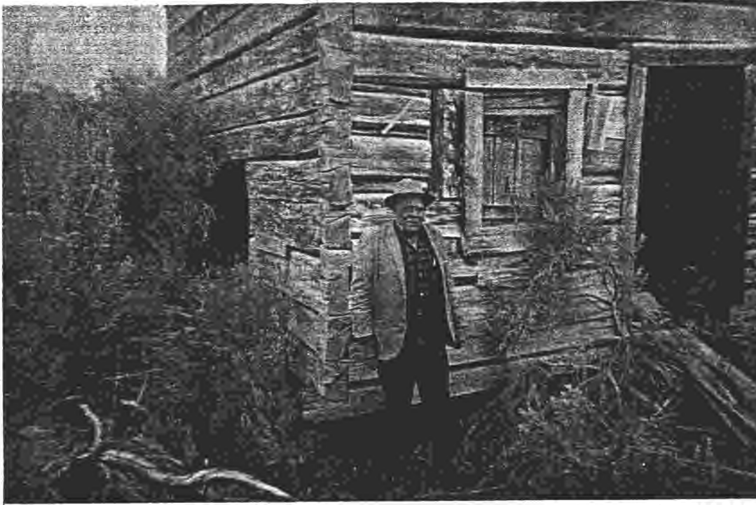
HOME WAS NEVER LIKE THIS! Rube Long surveys the cabin in which he spent a few of his early years on the High Desert. Interlocking hand-hewn logs have withstood nearly 90 years of sunshine and storm. Plans are now being considered for moving the ancient structure to nearby Christmas Valley for preservation and restoration.
