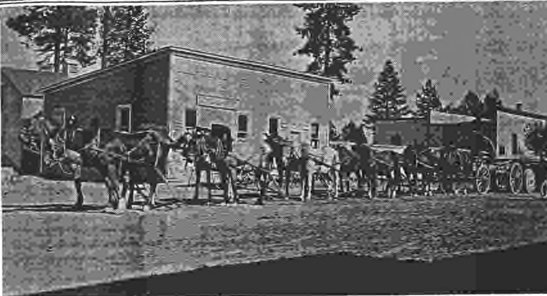
This picture was taken in 1910 on Oregon Avenue between Wall and Bond Streets. The occasion was the arrival of a turbine and large gear wheel for the first electric power plant at Bend. The team, owned by Jack Kelley and Ralph Dunn,
